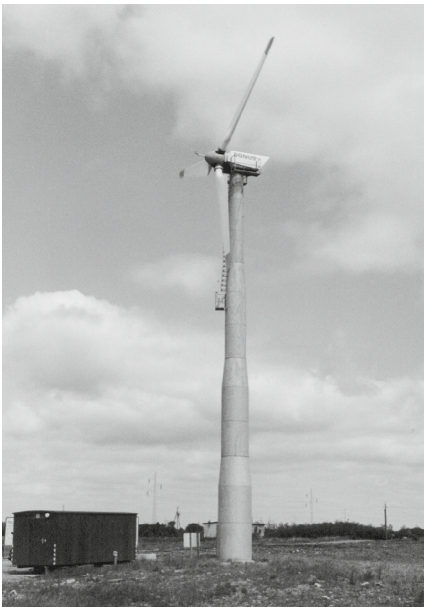
Fig. 12.5. Stepped tubular steel tower of a Bonus turbine (1985)
