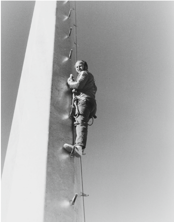
Fig. 12.18. Tubular-steel tower of a small wind turbine (Aeroman) that can be climbed from the outside
