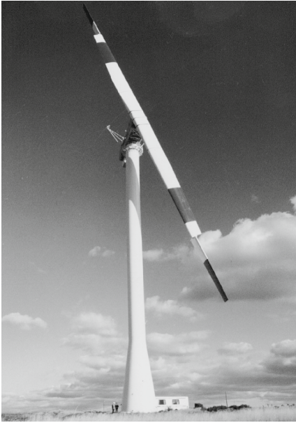
Fig. 12.3. Free standing tubular steel tower of the MOD -2 (1982)
