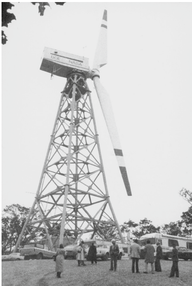
Fig. 12.1. MOD-1 with lattice tower (1982)
