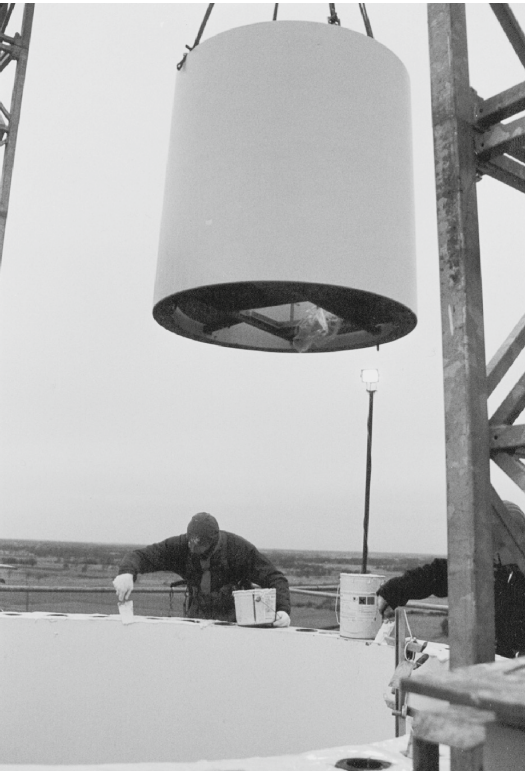
Fig. 12.25. Production of tower segments for a prefabricated prestressed-concrete tower (WEC-Turmbau)
