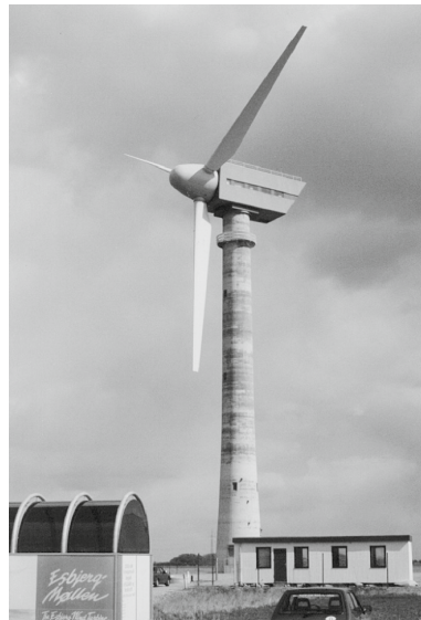
Fig. 12.2. Concrete tower of the Tjaereborg test turbine (1986)
