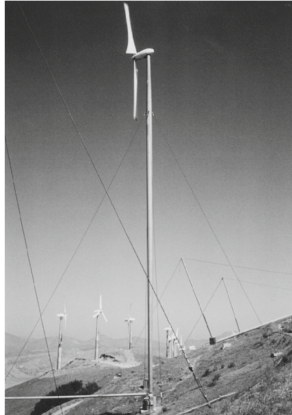
Fig. 12.4. Guyed tubular-steel tower of a Carter turbine (1985)
