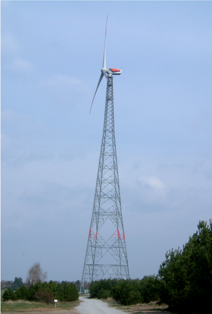
Fig. 12.21. Lattice tower of the Fuhrländer W2E (2.5 MW) with a height of 160 m (SeeBA)
