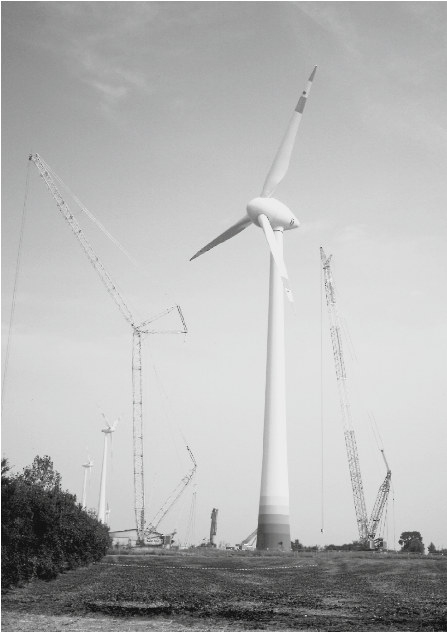
Fig. 12.23. Site-mixed concrete tower of the Enercon E-112 prototype, 120 m height
