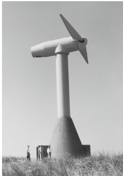
Fig. 12.6. Steel tower on a concrete base of the Dutch experimental turbine HAT-25 (1985)
