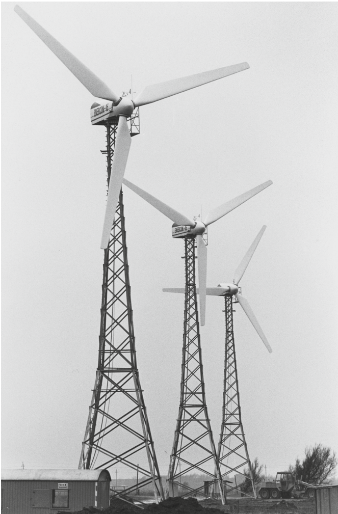
Fig. 12.19. Small wind turbines with lattice towers (1985)
