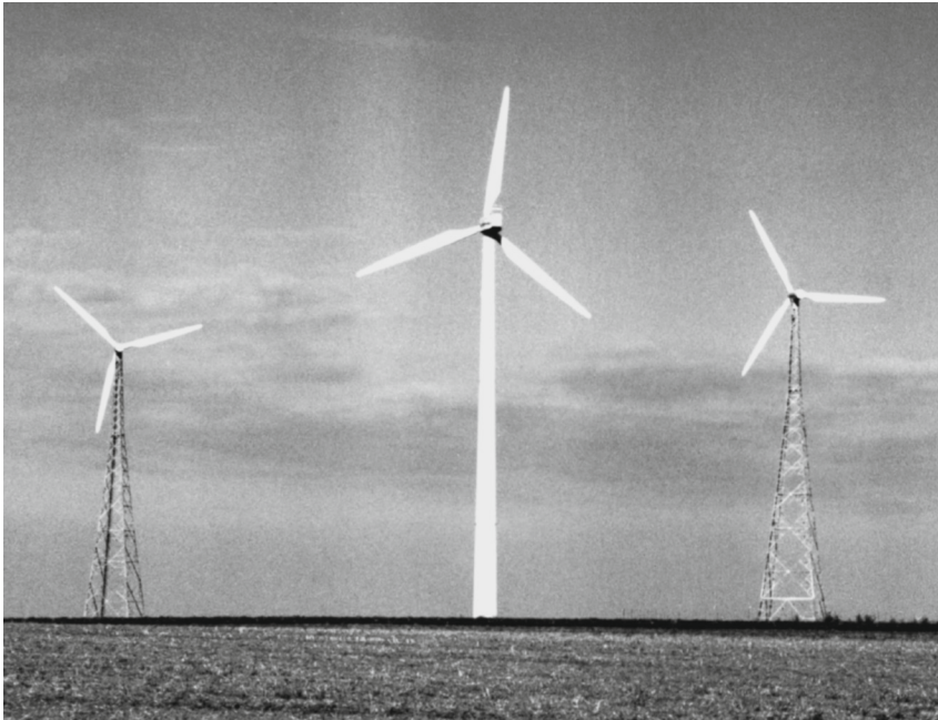
Fig. 12.20. Wind turbines with lattice towers and with tubular-steel tower (photo Sinning)
