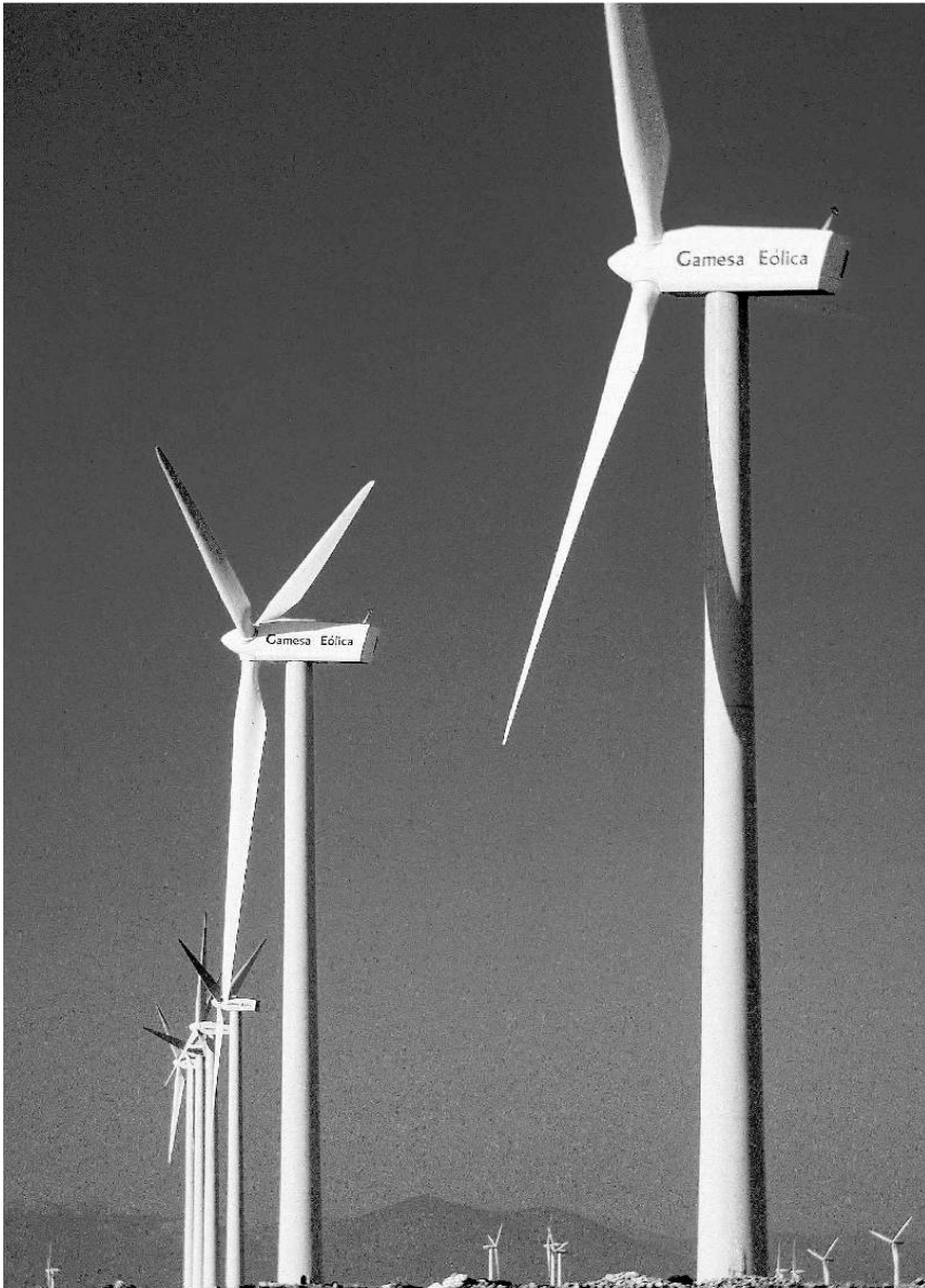
Fig. 12.8. Free-standing tubular towers of GAMESA wind turbines
