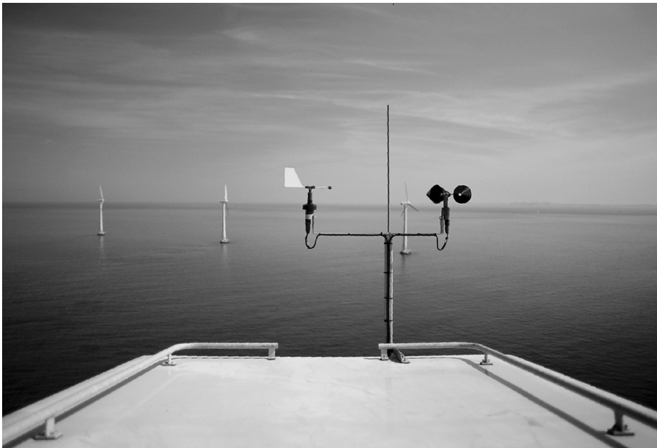
Fig. 11.2. Operational wind measuring system on the nacelle of a Vestas offshore turbine
