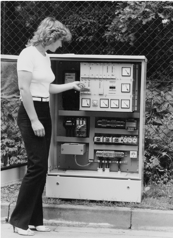
Fig. 10.39. Switchbox of a small Aeroman wind turbine
