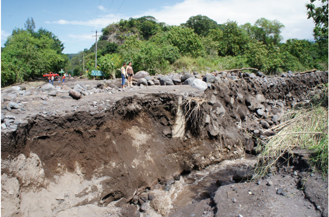
Fig. 7 Evacuation route damaged by a lahar. The community of La Becerrera, Colima, is surrounded by La Lumbre, El Zarco and El Cordobán rivers, which experience lahars during almost every intense rainfall event, with some of them affecting the communication routes. The image shows a road that serves as an
