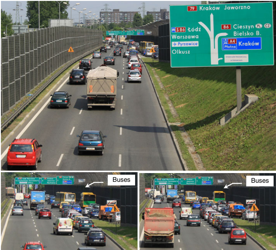
Fig. 6. Weaving section at the exit from the tunnel with flows in four directions – see road sign
