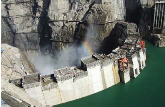
Fig. 10.16 Laxiwa Hydraulic Power Station on the Yellow River, China
