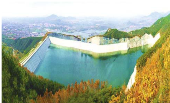
Fig. 10.29 Top water reservoir of the Tai'an Pumped Storage Hydraulic Plant
