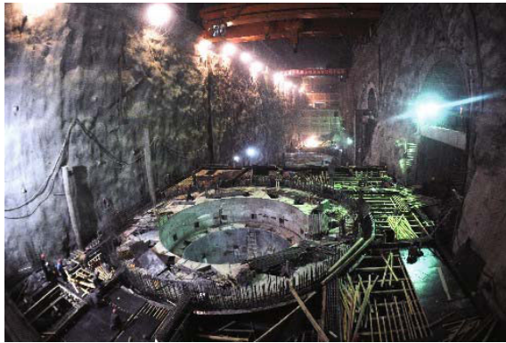
Fig. 10.17 Large cave of Laxiwa Hydraulic Power Station
