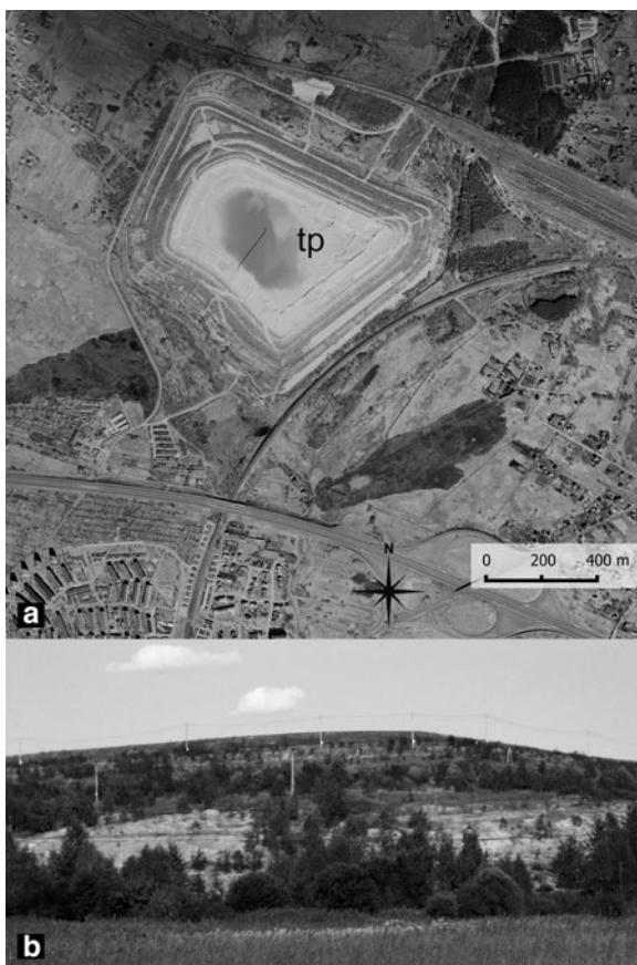
Fig. 16.1 Tailing pond of the ZG Trzebieńka industrial site: (a) aerial view on the tailing pond (tp); (b) tailing pond as seen from ground surface
