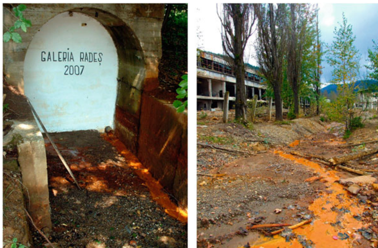
Fig. 3.3 Acid mine drainage from a closed mine gallery ( left ) and from closed tailing dam ( right )
