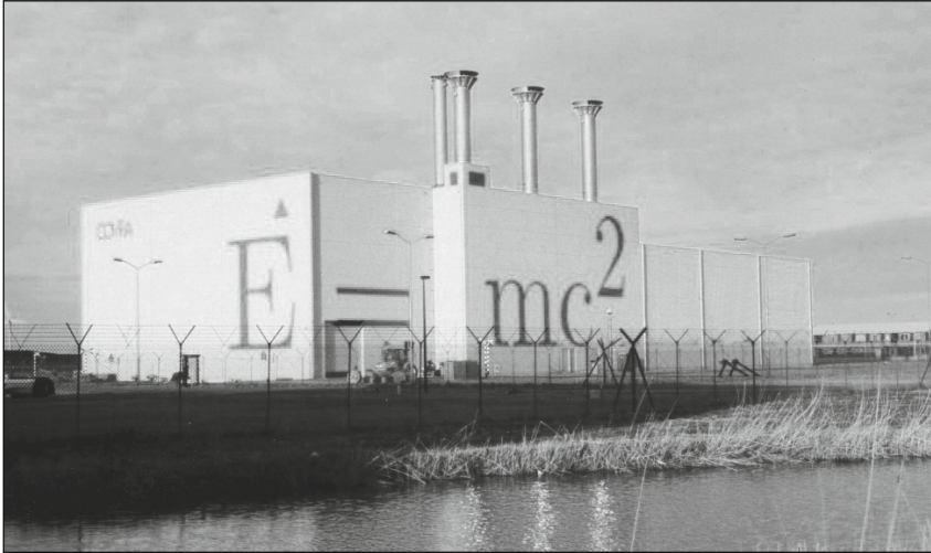
Fig. B.9: The HABOG storage facility in Zeeland (The Netherlands; photo: K.-J. Röhlig)
