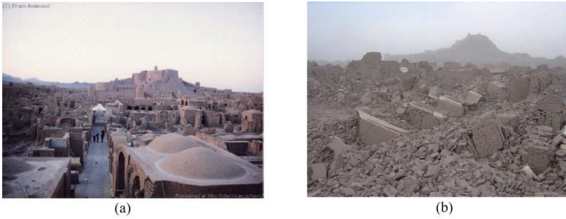
Fig. 1. Citadel of Bam : a view form the first city wall toward the bazaar, governor’s district and main tower (a) before the earthquake (b) after the earthquake
