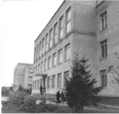
Fig. 2. Two of three buildings, from its beginning; Soviet Center of Microelectronics in Zelenograd
