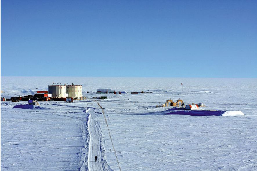
Fig. 32.1 Concordia station. The two principal towers can be seen; the ‘noisy’ tower which houses life support, recreation, food storage and preparation, and the mess; the ‘quiet’ tower which houses sleeping quarters, laboratories and medical
