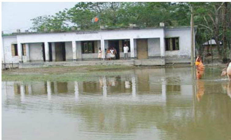
Fig. 12 An affected primary school in Keshabpur Upazilla . Source: Khan (2008)
