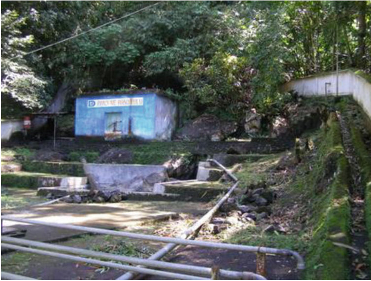
Fig. 3 Danowudu reservoir managed by PDAM and PAND
