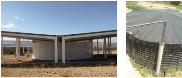
Fig. 2 Examples of rainwater harvesting tanks in Mexico. On the left : catchment and storage of rainwater for a small community (129 inhabitants) in Aguascalientes (Source: Aguascalientes 2006). On the right : rainwater harvesting tank in a state school, Estado de México (Source: Marth)
