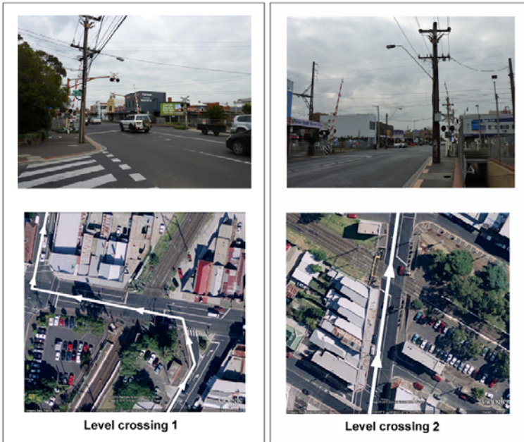
Fig. 2. Bird's eye and approach views of rail level crossings involved in study
