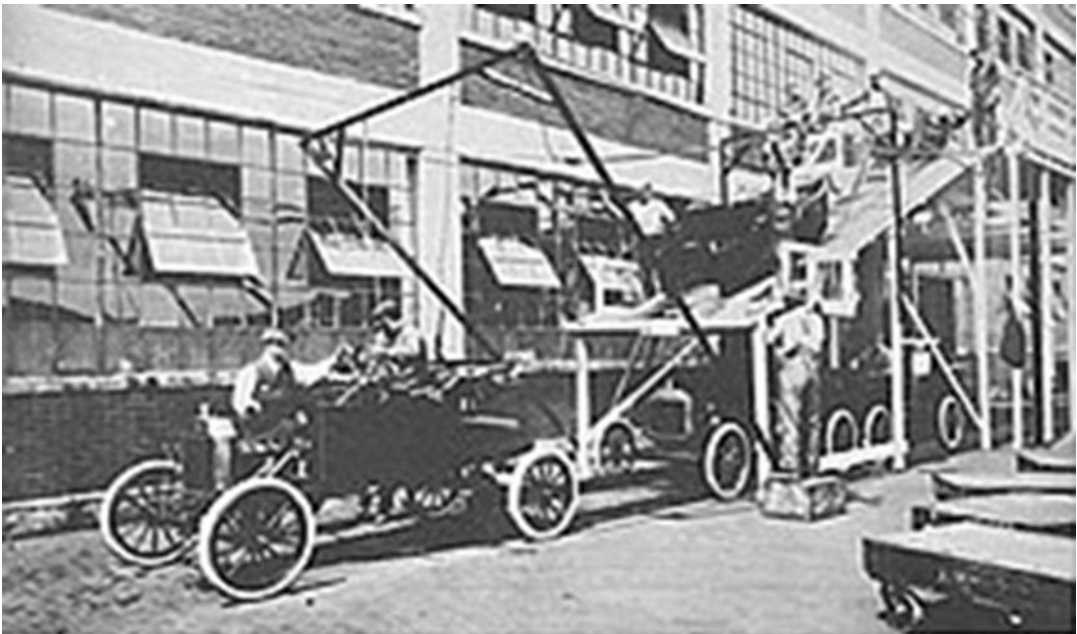
Assembly, Fig. 3 Henry Ford assembly line at Highland Park (Henry Ford 1908)
