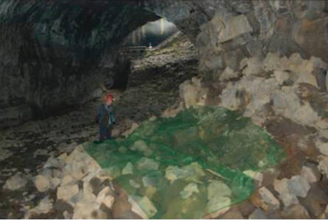
Fig. 10.3 Monitoring of rockfall in the lava tube cave near the road
