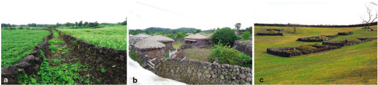
Fig. 6.79 Various types of Jeju Doldam (stone wall): Batdam as a field fence (a), Uldam as a fence of house (b), and Sandam as a graveyard fence (c)
