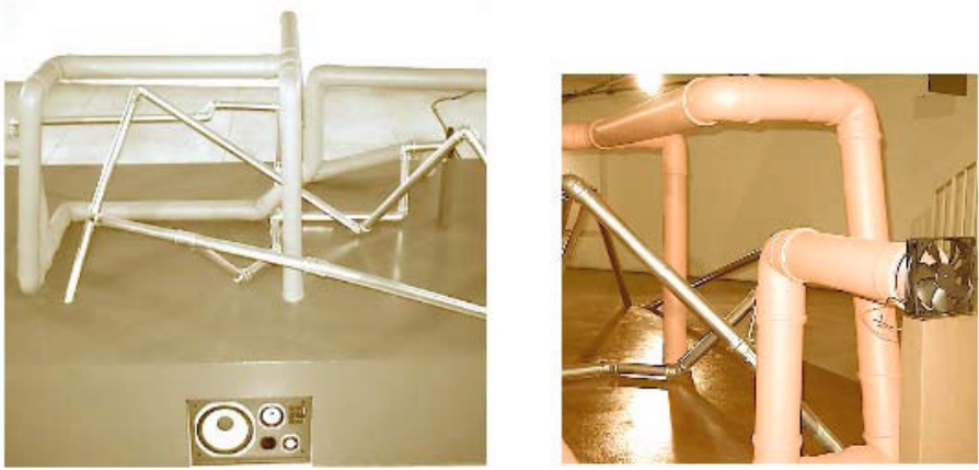
Fig. 1. Image of the VR installation. The plumbing structure (left), and a closeup of one fan attached to one of the vented ends of these pathways (right).
