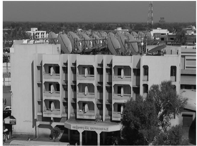
Figure 2: Installed Scheffler Concentrators, Project from 2001
