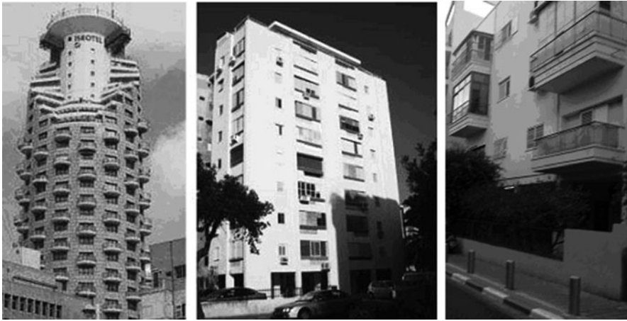
Fig. 15.1 Tel Aviv Balconies. Right: Typical Tel Avivian balconies of the 1950s and 1960s. Note that the balconies on the first floor of the building are “open”, while the others are “closed”. Center: Following the municipalities’ new rules, developers started to build buildings with closed balconies. Left: A building with “jumping balconies” Left and Center from Alfasi And Portugali 2009, Fig. 5
