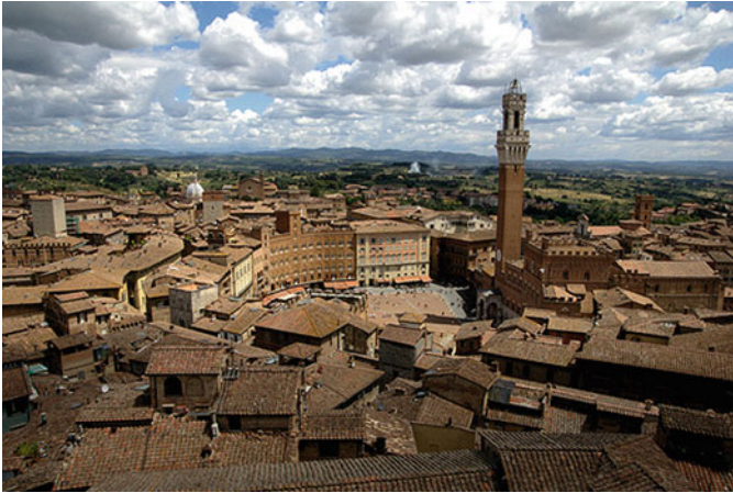
Fig. 8.12 The tower house of Piazza del Campo at Siena
