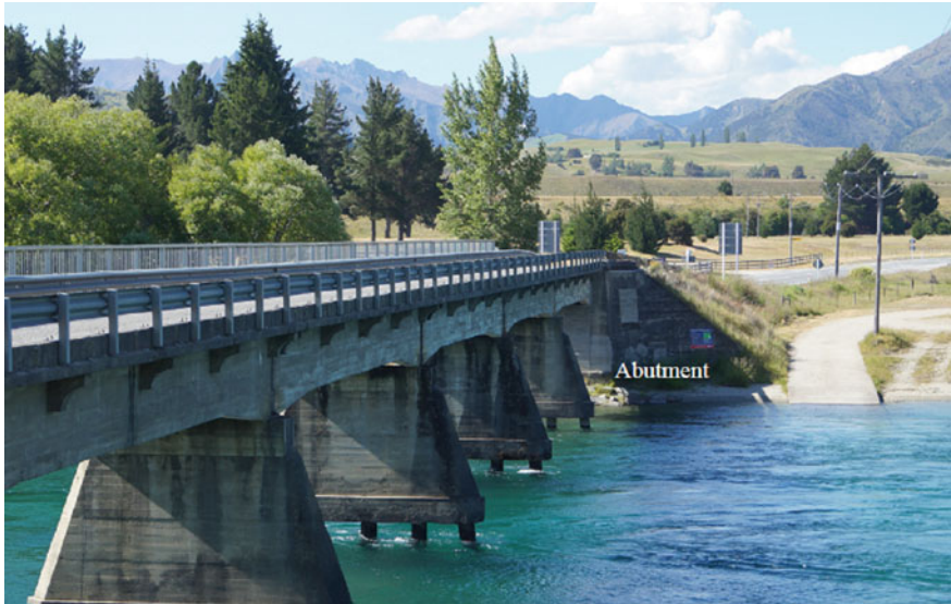
Fig. 10.23 Photograph of a wing-wall abutment. Photograph by the author
