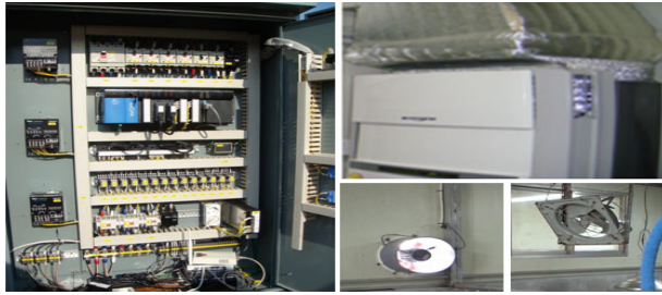
Fig. 4. Environmental control device and Pigpen facilities
