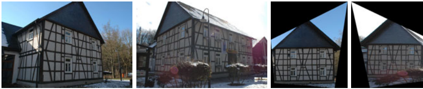
Fig. 2. Some examples of viewpoint normalization. Left: Original images; Right: Normalized front views. Note the perspective distortions are largely reduced in the warped front-parallel views of the building walls (e.g. a rectangular window in the 3D world will also appear rectangular in the normalized images).
