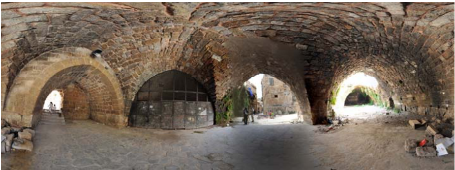
Fig. 5. Spherical panorama inside the vaulted galleries (Citadel of Tartous)
