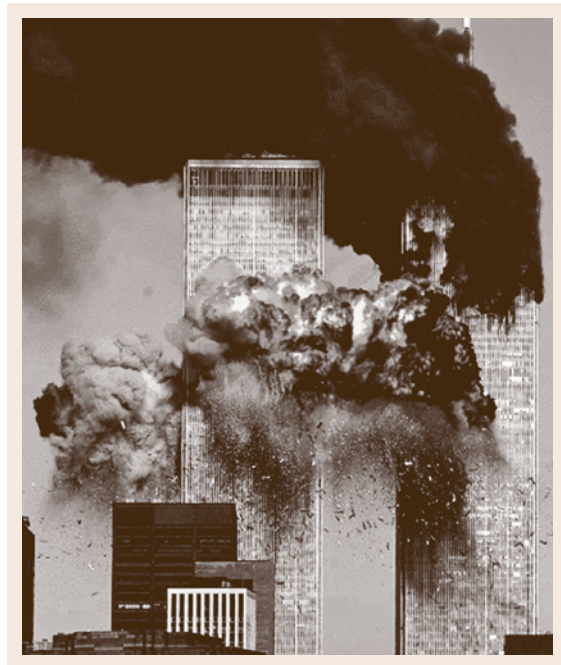
Fig. 15.34 The jet fuel started intense fires that caused the World Trade Center towers to collapse on September 11, 2001
