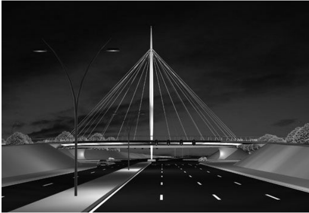
Fig. 5a. Footbridge for pedestrians and cyclists elevated over an intersection. Source: [7].
