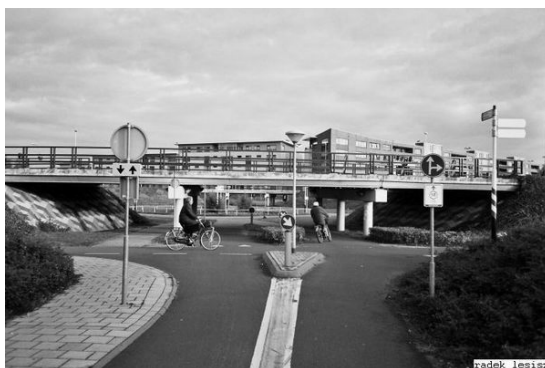
Fig. 6b. Sectioned bicycle paths under an elevated roundabout. Source: [4], [8].
