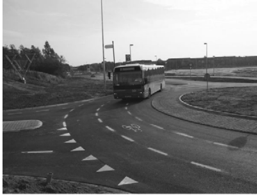
Fig. 8a. Roundabout with a bicycle path in the middle of the road. Source: [7], [8].
