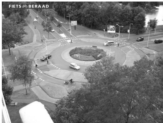
Fig. 3b. Roundabout with sectioned bicycle lanes. Priority given to the cyclists. Source: [7].
