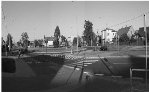
Fig. 4b. Roundabout with sectioned bicycle lanes. No priority given to the cyclists. Source: [6].
