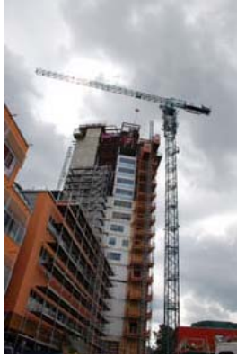
Fig. 1. Tornet (The Tower) during construction
