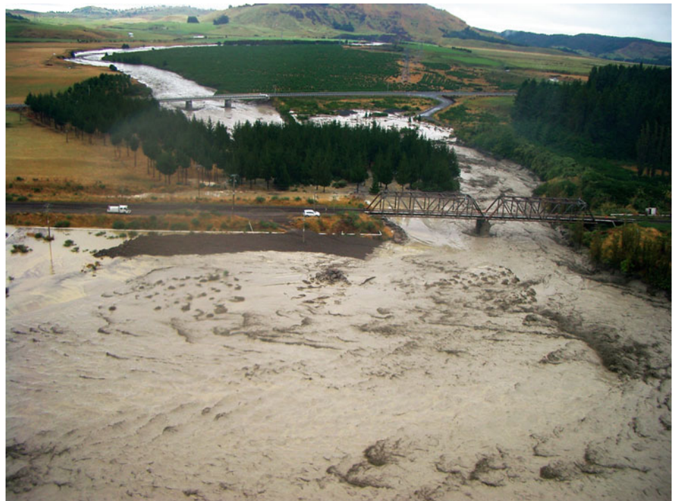
Fig. 12.17 Aerial view of the 18 March 2007 lahar at Tangiwai just after the flood peak, with the rail bridge in the foreground and the 1953 memorial area and highway bridge in the middle background. Six years later visible evidence of the lahar passage includes the concrete floor of a toilet block that was swept away, twisted cables of a safety barrier, sediments, and the newly exposed remains of the rear bogie of the locomotive involved in the 1953 disaster. Photo Harry Keys
