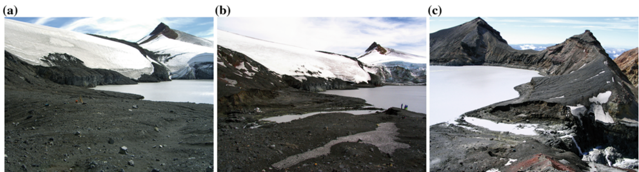
Fig. 12.16 a ( before breakout) b and c ( after breakout) showing the 60 m wide and 7.5 m high breach in the tephra dam created on 18 March 2007 and which released 1.3 million cubic metres of Crater
