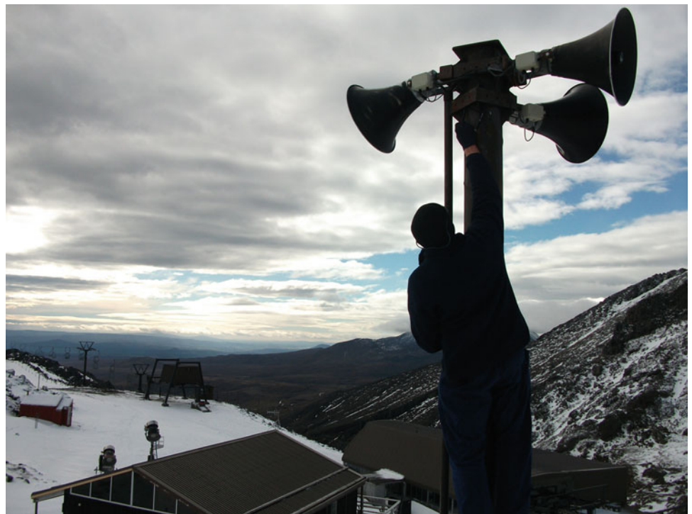
Fig. 12.29 When an eruption is detected EDS speakers on Whakapapa ski area broadcast sirens and pre-recorded messages warning people to move out of valleys in case a lahar is approaching. Photo Harry Keys
