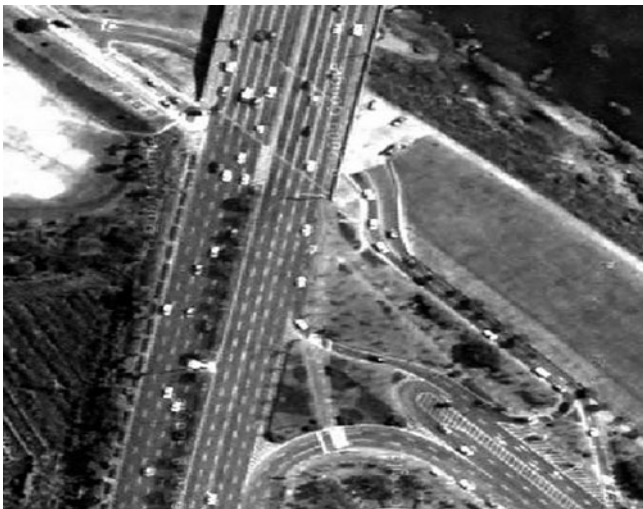
Fig. 4 Google Earth view of a unregulated intersection
