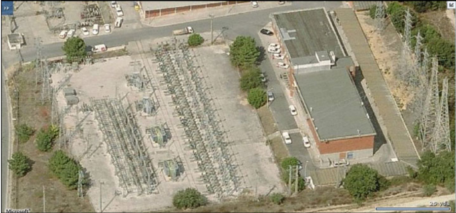
Fig. 3. Substation perimeter surveillance
