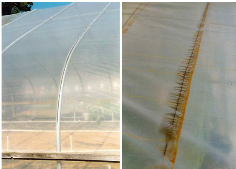
Fig. 8.26 Direct contact of the plastic film with steel tubes is a problem, in particular on hot days. The steel pipes can be heated up to 70°C by direct solar radiation. The plastic film can be destroyed earlier. In addition, the plastic film rubs on the steel tubes and the wires, and becomes black. This causes destruction of the film. It is recommendable to put some plastic tapes between film and steel pipes (Fig. 4.4). Another possibility is to paint the plastic white at the contact point to the steel pipes to prevent them from becoming too hot
