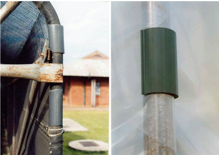
Fig. 8.18 Self-made clips for fastening of film or nets. One can use pieces of plastic water tubes which are cut open in a longitudinal direction and put over the construction component with the film or net in between, if no commercial fastening clips are available. This can be done even with timber profiles
