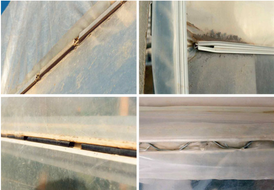
Fig. 8.21 A special method for fastening the film is to push the film into steel profiles using plastic profiles, spring steel or even rubber or plastic tubes
