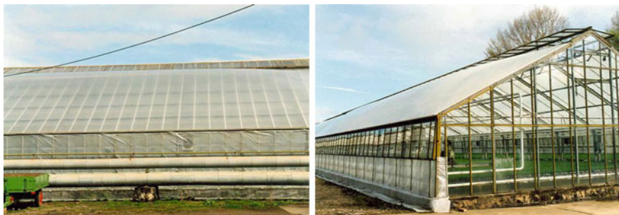
Fig. 8.25 Double-inflated film can also be used to repair and to use old structures, for example old glass houses. The old cladding material will be removed and double-inflated film installed
