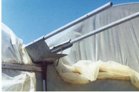
Fig. 8.19 Fastening and stretching of plastic film by rolling it up on a tube in the gutter. Either the gutter is formed especially for this reason, or a special holder can be fixed in the gutter. The sharp edges of the gutter should be protected by small plastic profiles to prevent cutting of the film. The advantage of this method is the fastening and stretching of the film at the same time
