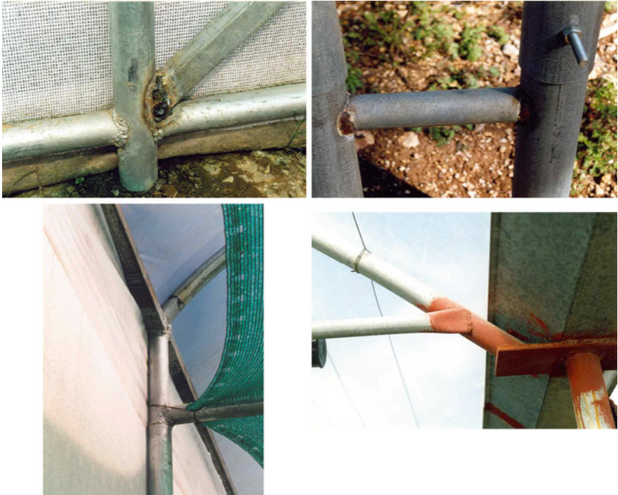
Fig. 8.11 Galvanised steel components welded together (see Sect. 8.2.1.1)
