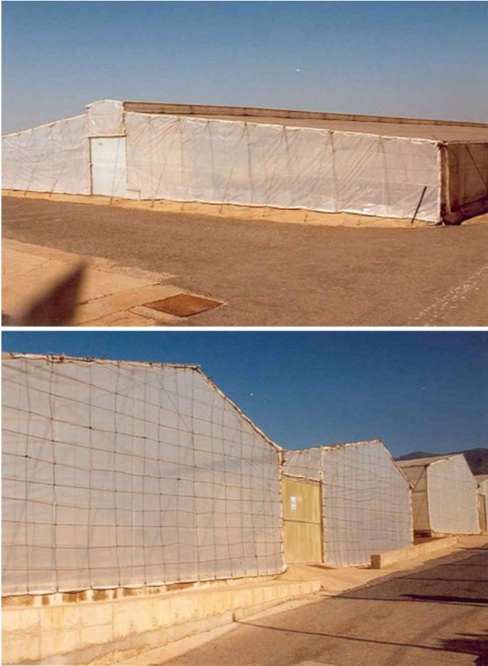
Fig. 5.72 The Parral-type constructions were improved to asymmetrical saddle-roof types with different roof slopes
