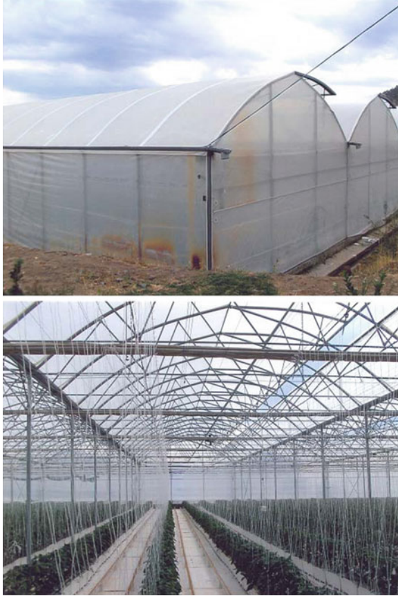
Fig. 5.22 Multi-span pointed-arched greenhouses with flap ventilation in Turkey. Thermal screen and hydroponic system inside
