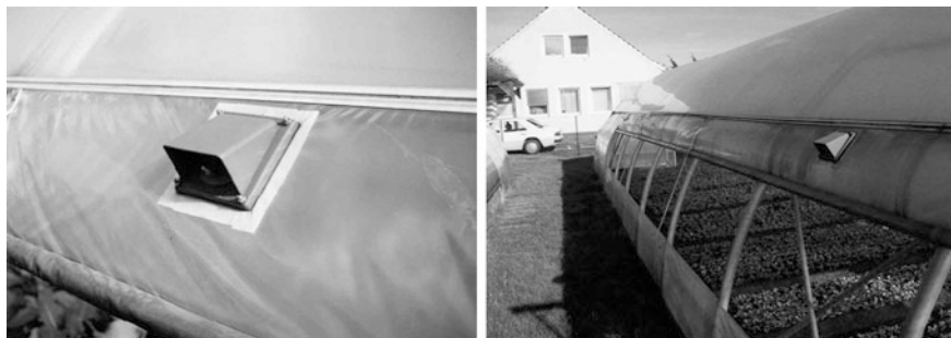
Fig. 5.85 Meanwhile, commercial valves for the double-inflated film are available
