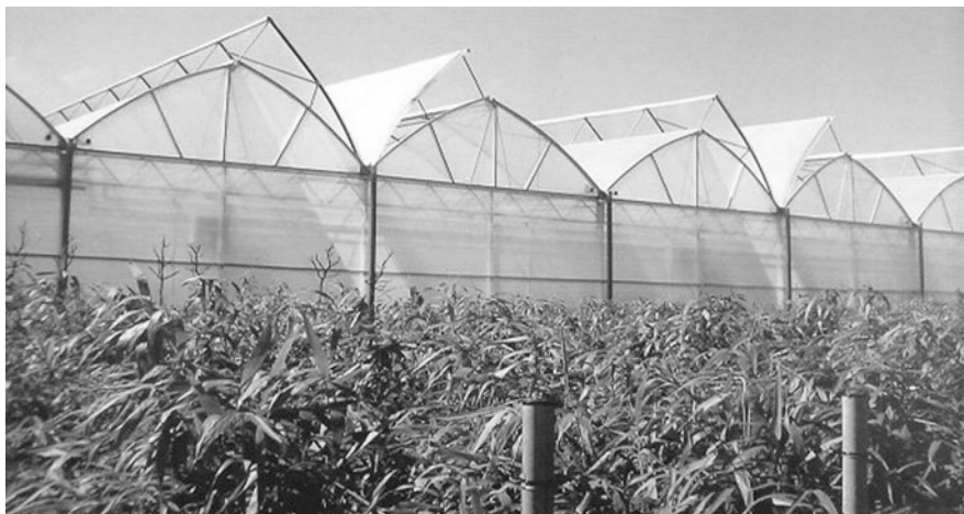
Fig. 5.55 Greenhouse structure with alternate roof openings. The roof opening is linked to the gutter, and opens at the ridge. The height of the gutter is more than 4 m
