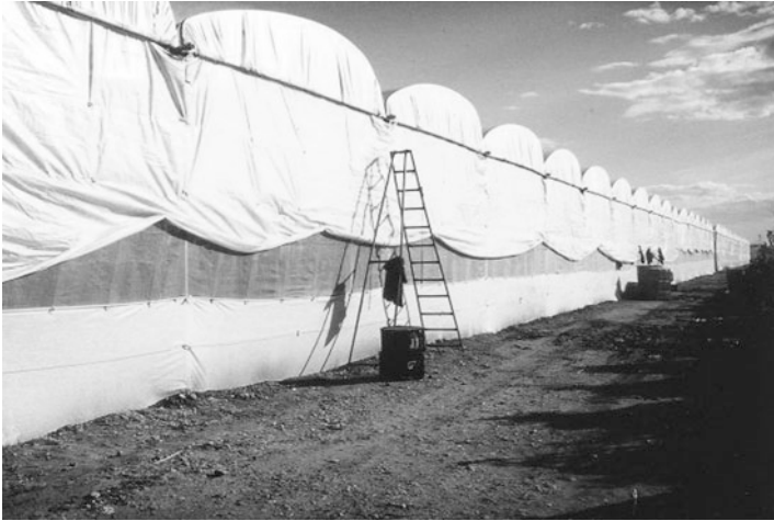
Fig. 5.47 Multi-span greenhouse in Morocco. The ventilation opening may be not sufficient
