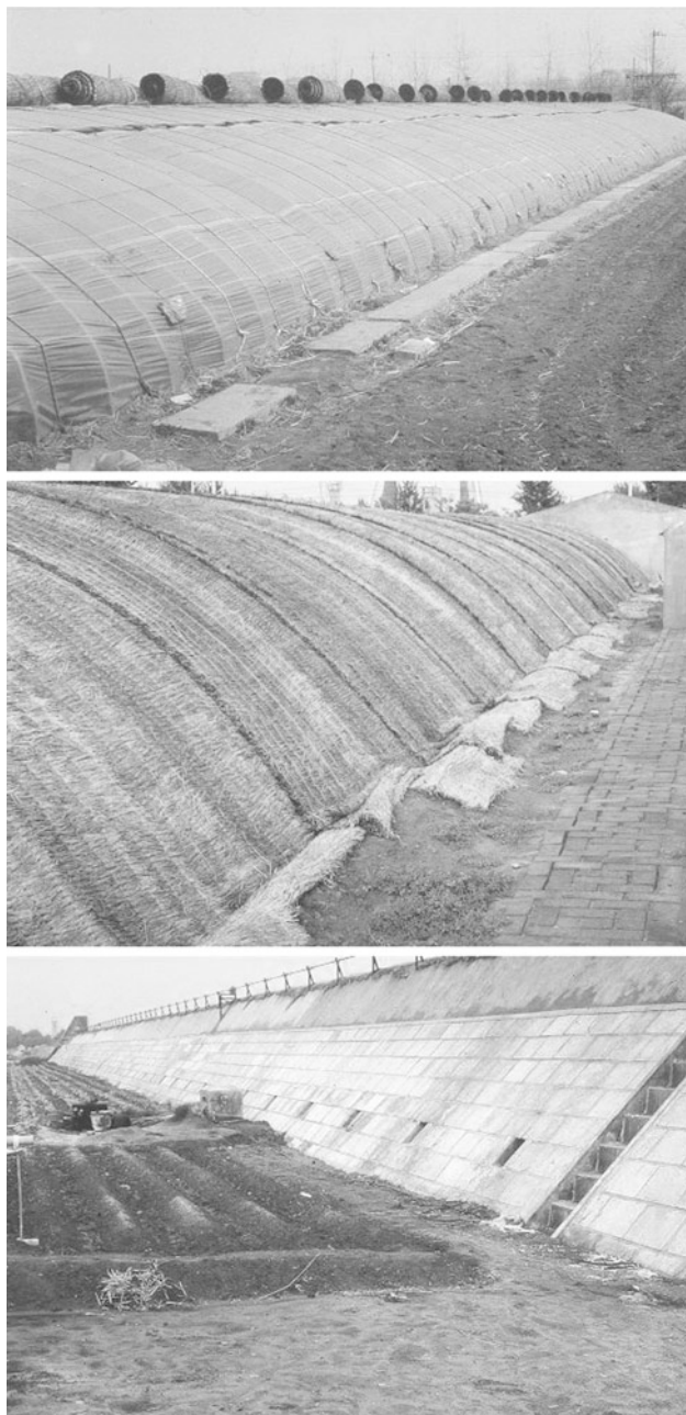
Fig. 5.56 Greenhouse in China. A round-arched structure is leaned against a north wall, and will be covered by straw mats at night
