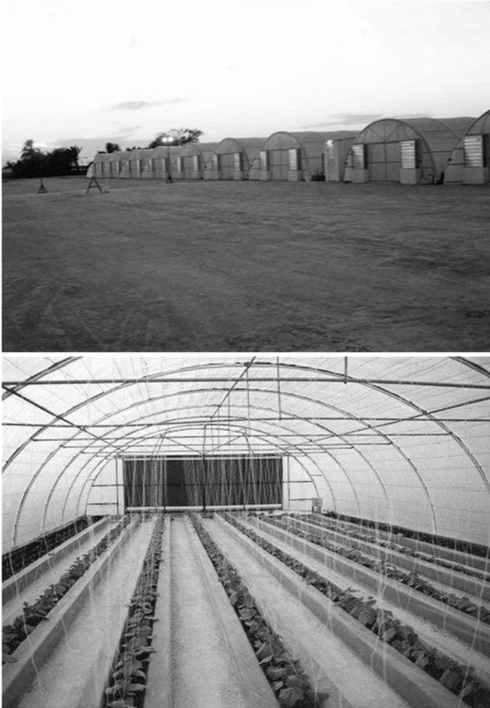
Fig. 5.62 Round-arched tunnel greenhouses with fan and pad cooling and hydroponics in the desert of Qatar
