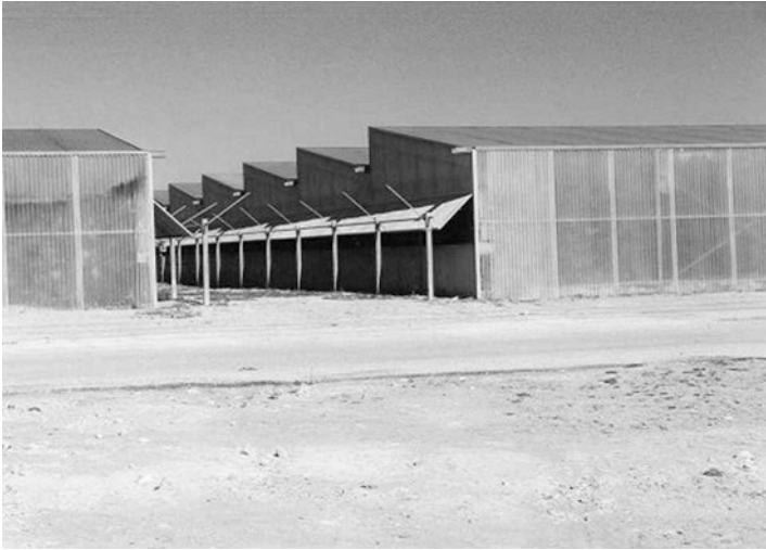
Fig. 5.63 Shed roof structure covered with corrugated polyester sheets. Those sheets are not recommendable anymore, because the light transmittance decreases within a short time and the sheets are relatively expensive.
