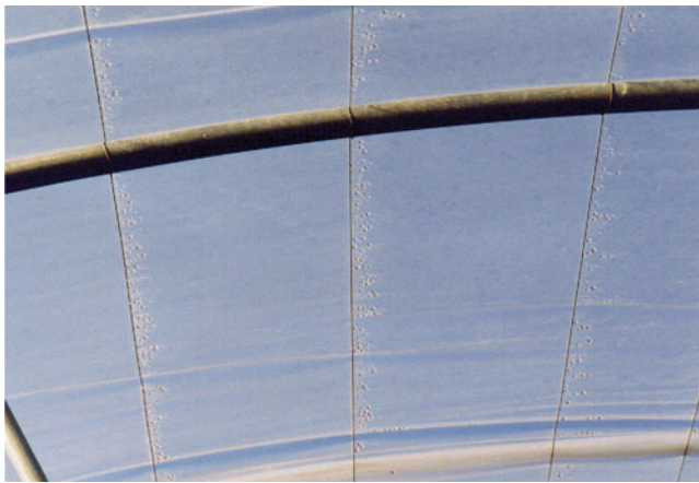
Fig. 5.5 Drop condensation at wires
