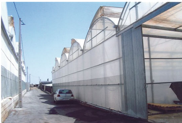
Fig. 5.73 Industrial manufactured high-arched greenhouses are used in particular for flowers
