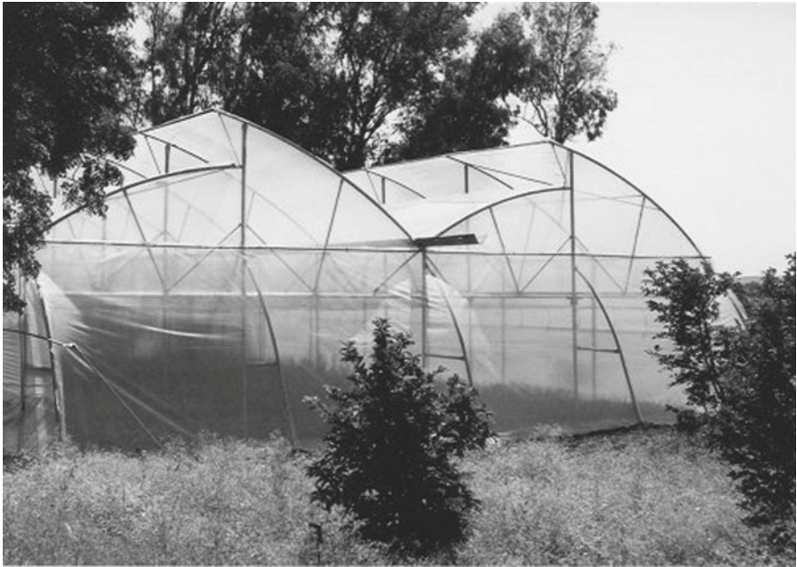
Fig. 5.40 Very stable steel tube structure from India, with bent roof and side wall tubes
