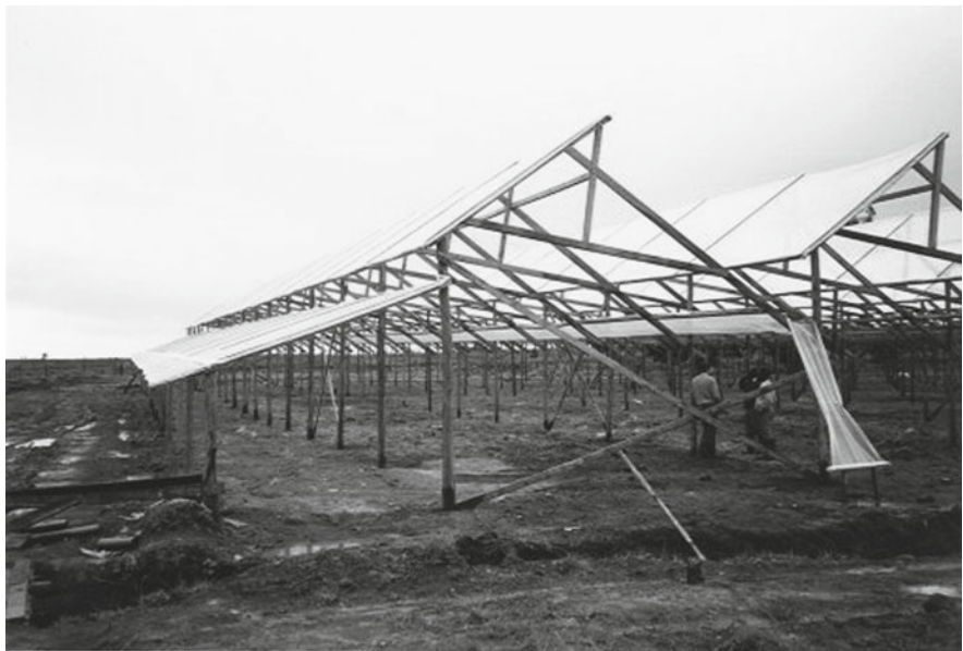
Fig. 5.35 Wooden structure from Kenya: 6.4 m ridge height, high volume and a canopy for rain protection on the weather side. The plastic film gutter is not advisable because of getting water pockets. The canopy at the side wall against sloping rain fall is highly recommendable
