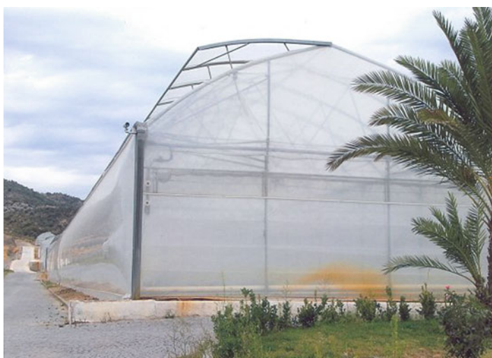
Fig. 5.54 Greenhouse with flap ventilation and high side wall in Turkey. The side wall is double-inflated
