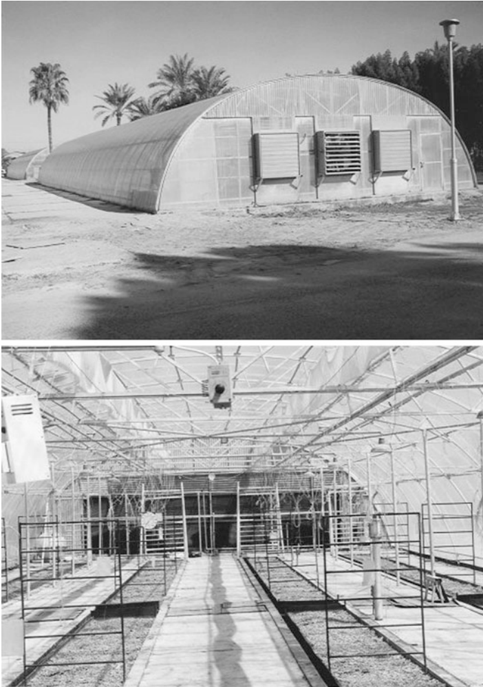
Fig. 5.60 Round-arched tunnel with fan and pad cooling at gable ends in Kuwait
