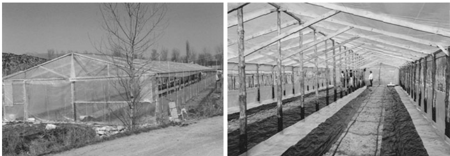
Fig. 5.44 A well-designed wooden structure in Albania
