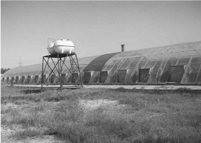
Fig. 5.61 Round-arched tunnel with fan and pad cooling at side wall in Kuwait
