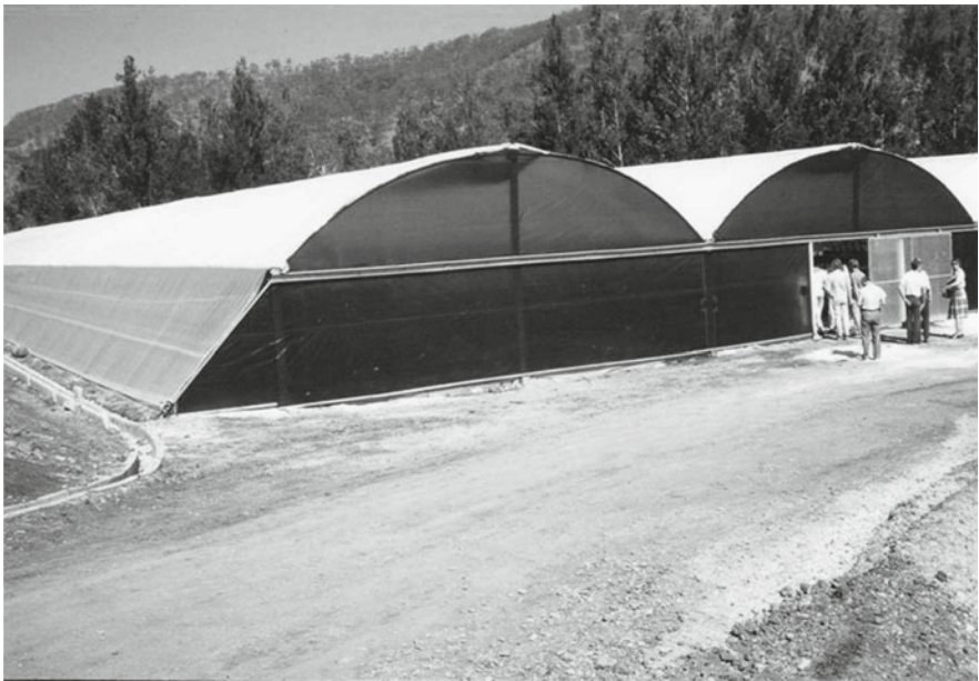
Fig. 5.87 Australian design with inclined steel ropes at the side walls for stabilizing the structure. The plastic film will be rolled up at the inclined ropes for ventilation. The gutters and steel tubes inside the greenhouse are connected and guyed by ropes
