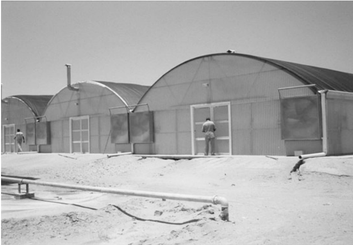
Fig. 5.58 A round-arched structure covered with plastic film and permanent shading net, ventilated and cooled by fan and pad system
