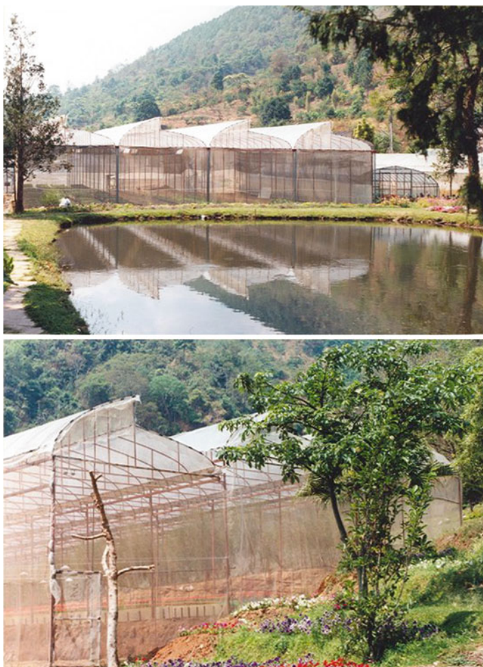
Fig. 5.38 Steel tube structure in Thailand with 5 m gutter height, ridge ventilation and nets against birds
