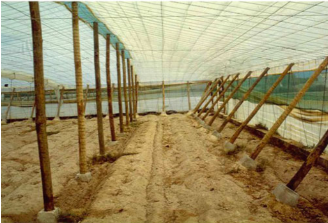
Fig. 5.68 Parral-type greenhouse in Almeria with flat roof
