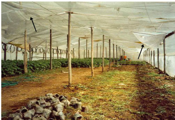
Fig. 5.71 Water pockets in the plastic film of flat roof
