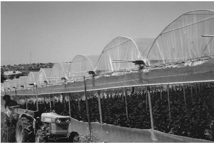
Fig. 5.48 Multi-span structure with roll-up ventilation in Cyprus
