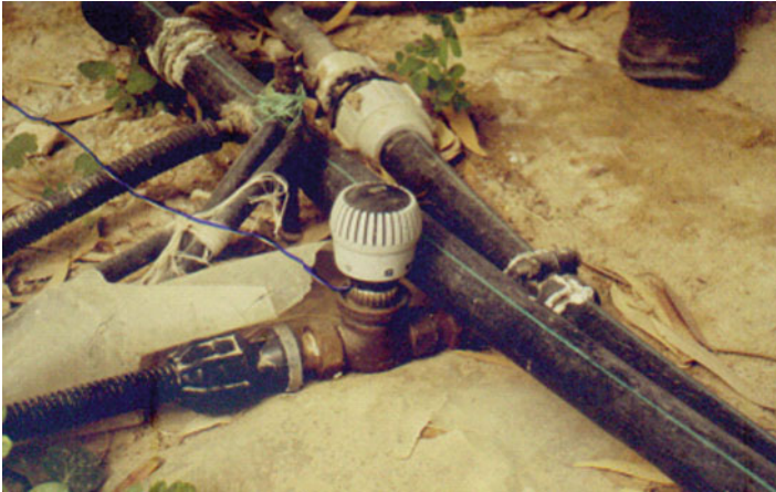
Fig. 12.16 Simple control system by thermostat
