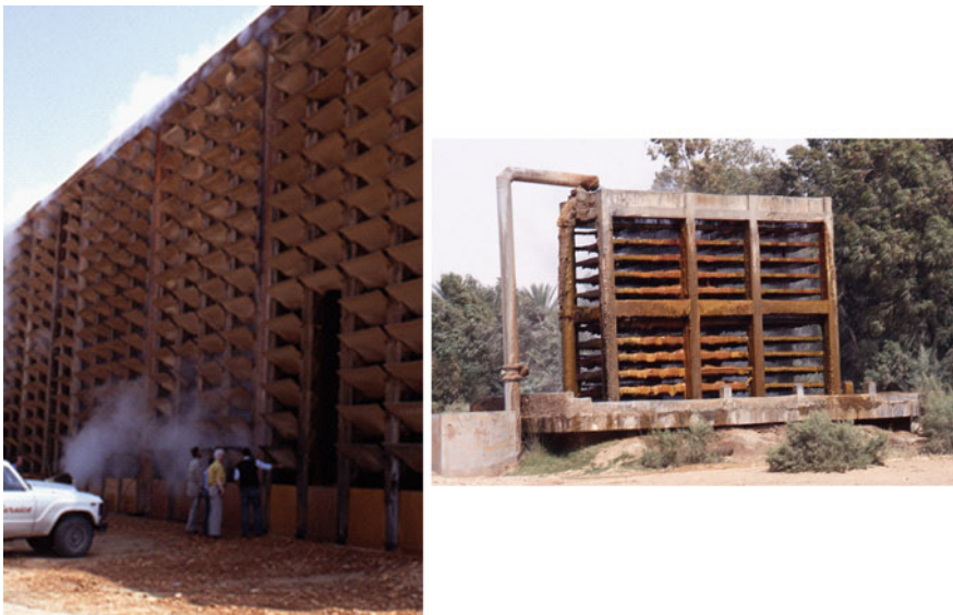
Fig. 12.12 Cooling towers to cool geothermal water for irrigation in Tunisia
