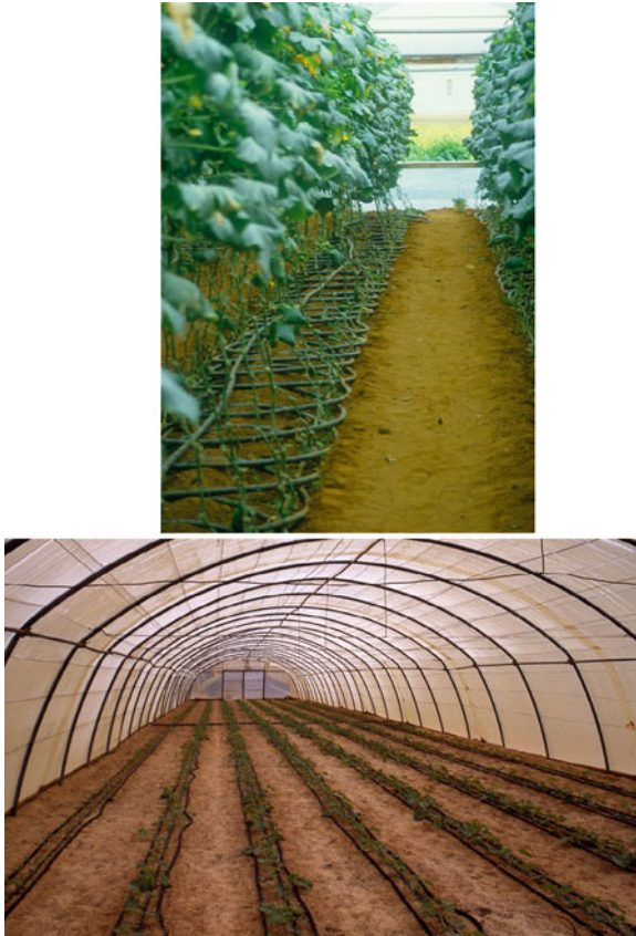
Fig. 12.10 Corrugated plastic tubes for greenhouse heating
