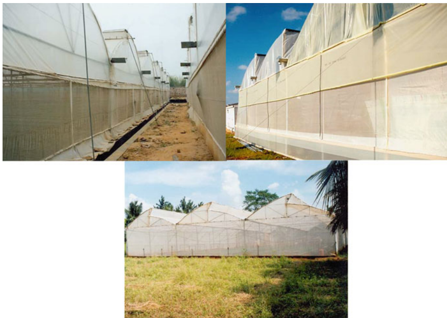
Fig. 10.14 Very well-installed and fixed insect screens at side walls and ridge ventilators
