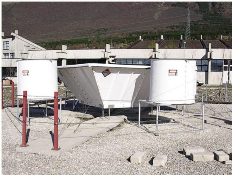
Fig. I.4.6 Picture of the wind profiler – RASS system located on the top of one building of the National Laboratory of Gran Sasso (LNGS), at an altitude of 981 m ASL. It works at 1,290 MHz, relative to a wavelength of about 23 cm
