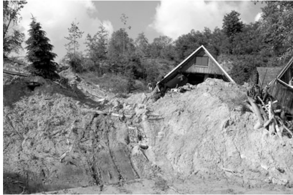
Fig. 1 Landslide activated by a heavy rainfall in May 2010 destroyed houses and agricultural land on the slopes of the Wieliczka Foothills, Polish Carpathians, at Winiary
