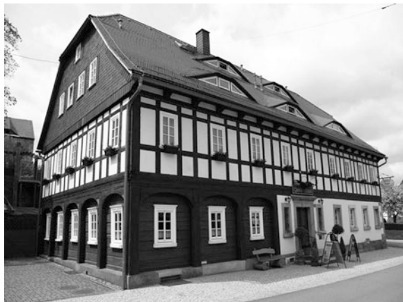
Fig. 8 Typical folk architecture in traditional weaver villages of Upper Lusatia (Saxony, Germany). Special efforts are necessary to maintain such nice old houses (Photo: O. Bastian)
