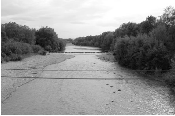
Fig. 2 Following straightening, considerable narrowing and partitioning by a number of concrete weirs, the contemporary Czarny Dunajec River in its channelized reach exhibits poor hydromorphological quality (Wyźga et al. 2010), reflected in degraded fish and benthic invertebrate communities. As many previously channelized reaches of Polish Carpathian rivers run through riparian forest, far from settlements and infrastructure, further maintenance of the channelization schemes is unjustified and there are no constraints on restoration of these reaches
