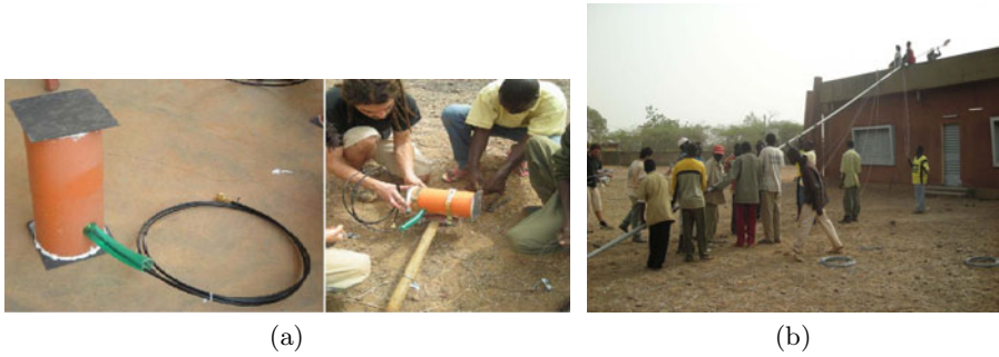
Fig. 4. (a) The antenna with a PVC radome ready to be installed; all the material is low-cost, recycled and locally available; (b) The set up of an antenna mast made by water pipes (third expedition, Jan. 2007)
