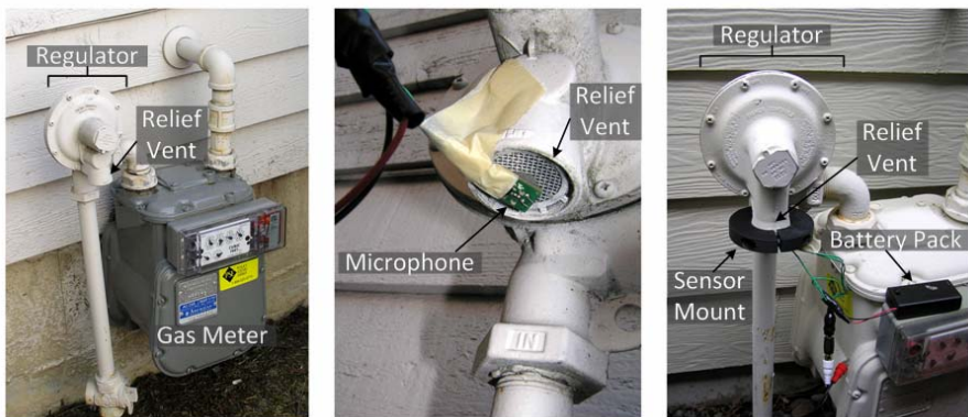
Fig. 1. (left) A typical US gas meter and pressure regulator. (middle) The location of our microphone-based sensor on the pressure regulator relief vent. (right) The GasSense prototype and sensor mount attached to the relief vent.
