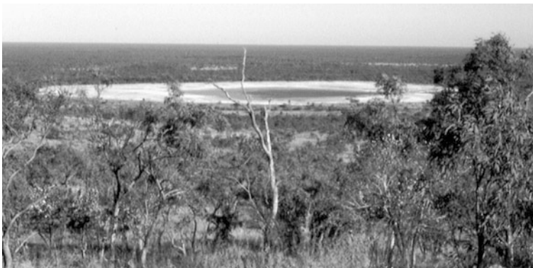
Fig. 4.7 Ponding of acid, saline water on an abandoned sulfidic tailings dam, Croydon gold mine, Australia
