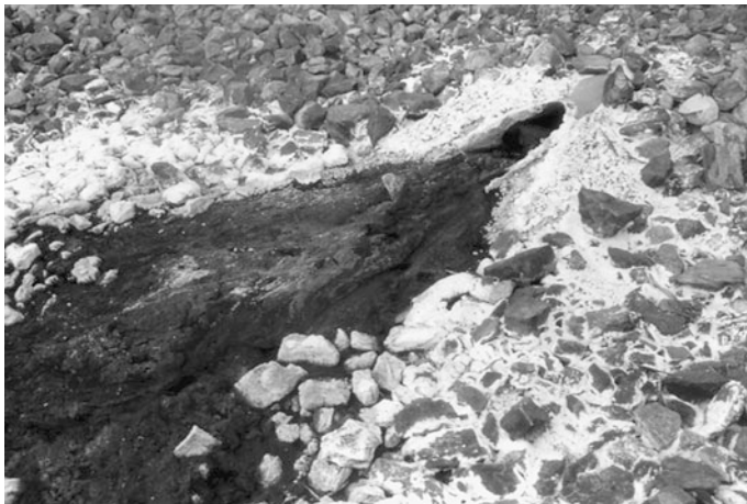
Fig. 2.26 Scalded seepage area at the base of White's waste heap (Fig. 2.25). The clay seal has cracked, and water infiltration into the dump has increased since the installation of the cover in 1984. Saline, acid seepages emanate from the base of the dump and precipitate abundant sulfate and iron oxyhydroxide efflorescences
