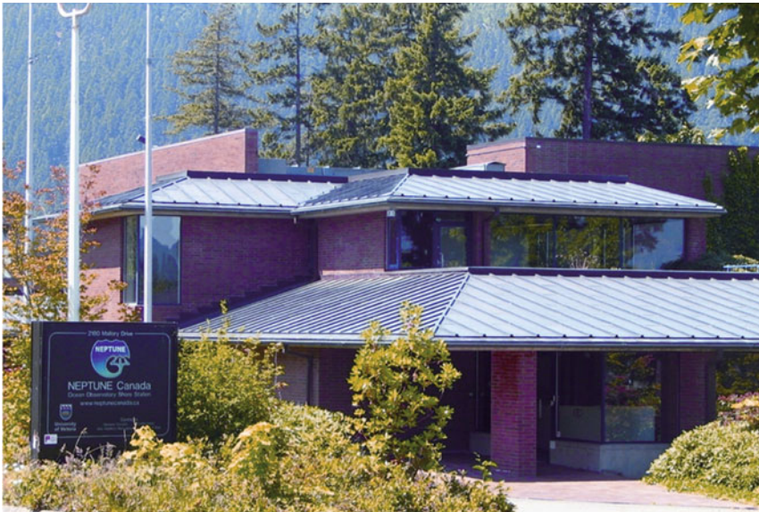
Figure 16.2 Shore station at Port Alberni.
