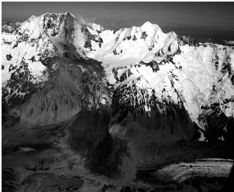
Fig. 17.3 The east face of Mount Cook collapsed in December 1991 releasing an avalanche of 12 \times 10^6 \text{ m}^3 of rock and ice. Based on seismogram (Fig. 17.4) interpretation, the bulk of the rock mass broke from the source in the first 20 s of the rapidly escalating collapse, and almost all of the mass was in simultaneous motion. Photo by Lloyd Homer
