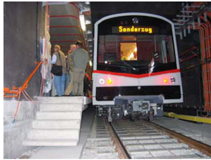
Fig. 5. Position of the side handrail and the stairs leading from the tunnel onto the platform of a station.
