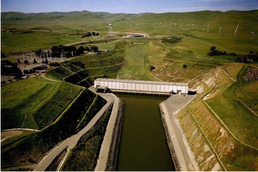
Fig. 2 The Harvey O. Banks pumping plant, which pumps Delta water into the California aqueduct, is shown. The plant can pump up to \sim 300 \text{ m}^3/\text{s} and lifts the water about 73 m to begin the transit southward through the 710 km of canals, tunnels, and pipelines that constitute the California aqueduct
