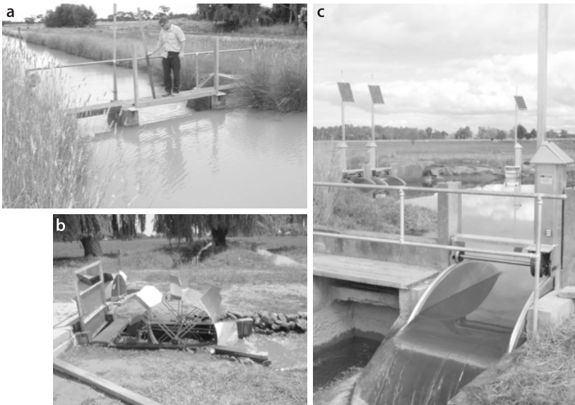
Fig. 3.4. Radio networked actuator/sensors for irrigation, developed in Australia by Rubicon Systems Australia, in collaboration with the University of Melbourne (c) replacing the old manually operated infrastructure (a–b)
