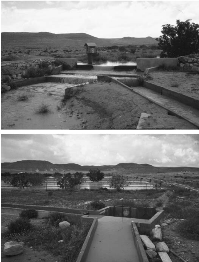
Fig. 21.10 Reconstructed runoff-rainwater farm at Avdat in the Negev desert after a rain in the spring of 1971 (original photographs Detlef Schulze)
