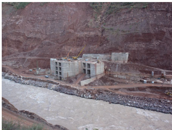
Fig. 9.3 Rogun dam site on the Vakhsh River, Tajikistan (Source: http://www.flickr.com/photos/32828146@N06/page10/ )
